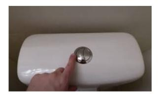
Alternatively, Top Flush toilets can have a single flush button (thus making them single flush toilets).
