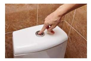
Single flush toilets are the most common type of toilet found in older homes and buildings. They have only one flush mechanism—meaning that all types of waste are flushed with the same amount of water.
